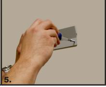
Mark the places where you will secure the plate. Using the marks made as a guide, fasten the tri-wall anchors. Mount the wall bracket onto the wall using the tri-wall anchors as guides. To secure the plate, attach the screws securely into the anchors.
